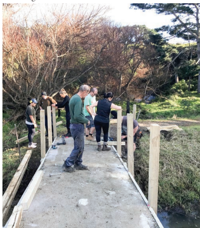
The working bee at Otahi Bridge on July 24, putting sides on the bridge upstream from the Otahi Road bridge.
